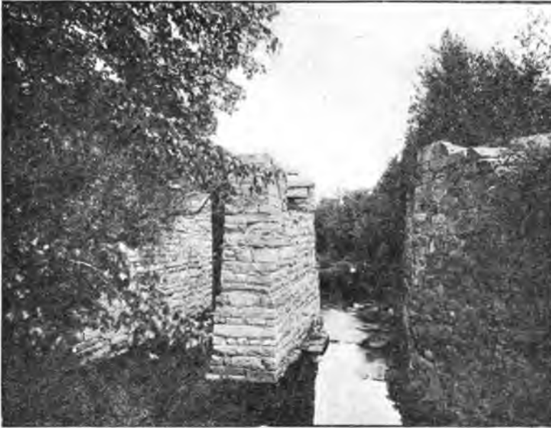
RUINS OF THE VIADUCT OVER SHAWSHEEN RIVER— MIDDLESEX CANAL, 1735.
